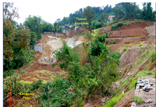
Figure 20d Collapse of anchored soil wall 31 st May 2006
