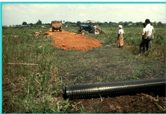
Figure 7 Laying of geogrid in soft ground
