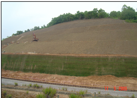
Figure 18f View of rehabilitated slope
