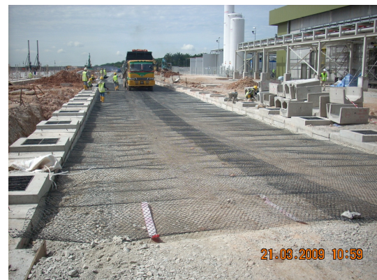
Figure 5d Laying of TriAx geogrid at Q-Cell in progress, 2008/2009
