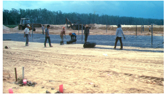
Figure 4e Muar Flat Trial 1987, laying of geogrids
