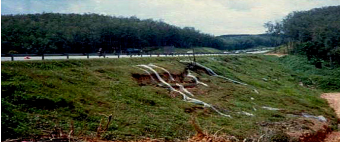
Figure 10a Picture of embankment failure, 1989.
