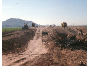
Figure 4b Excavation in embankment
