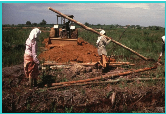
Figure 6 Laying of bakau mats for soft ground stabilization
