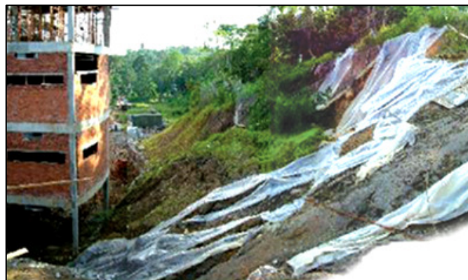
Figure 16a Slope failure affecting the lecture block
