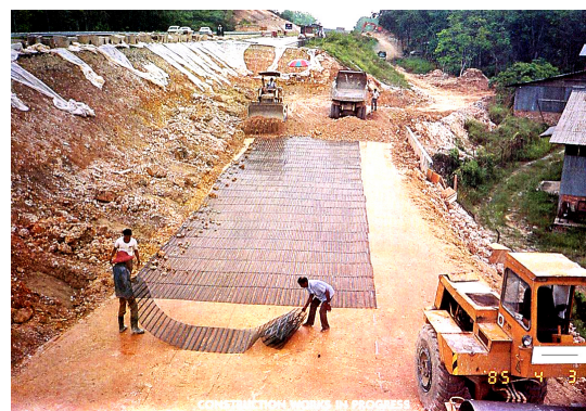
Figure 3b Rehabilitation in progress; laying of geogrid
