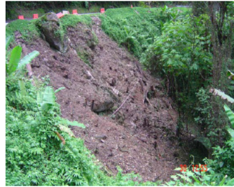
Figure 19a Collapse of embankment
