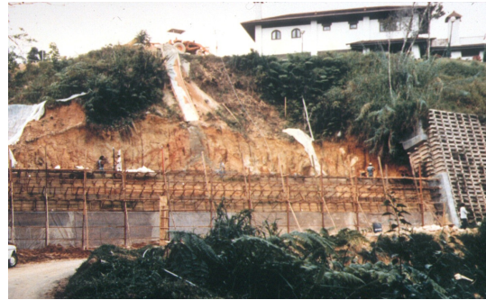
Figure 2a Petronas bungalow with failed slope in 1987
