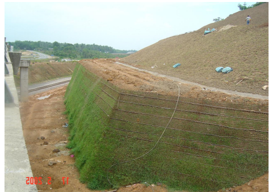
Figure 18e Turfing of geogrid block
