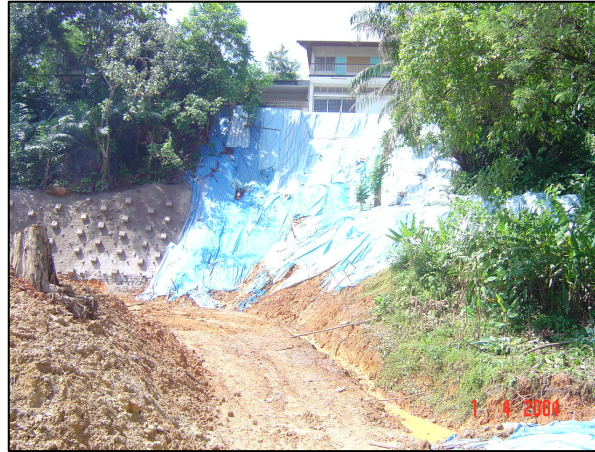
Figure17a Collapse of cut slope during soil nailing
