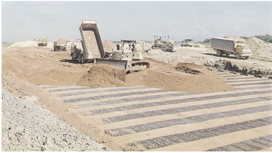
Figure 4d Laying of SR2 uniaxial geogrid
