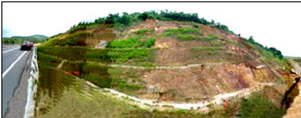
Figure 18a Overview of cut slope failure
