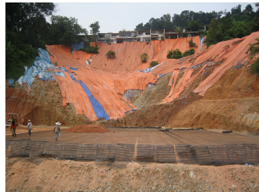
Figure 20i Construction of upper geogrid embankment
