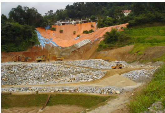
Figure 20h Construction of lower rock fill embankment
