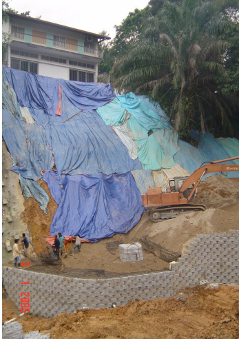
Figure 17d Construction of Modular Block wall with geogrid.
