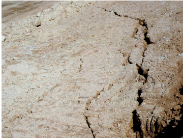
Figure 4a Crack in embankment
