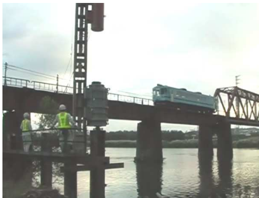
Photo 2 SH test beside the railway bridge in service
