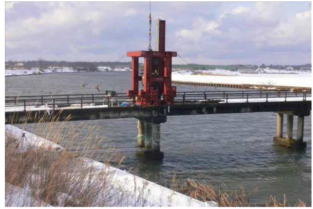
Photo 4 SH devices placed on the bridge
