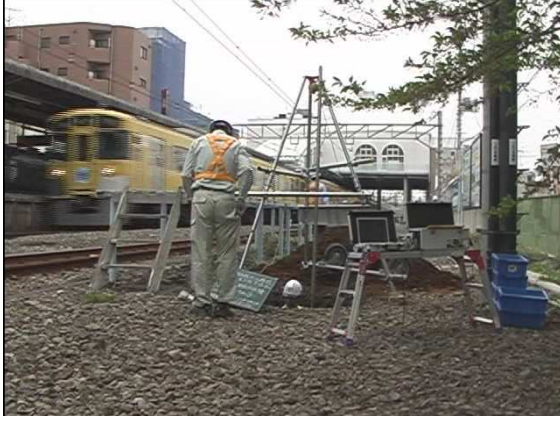
Photo 1 SH testing in the railway station yard
