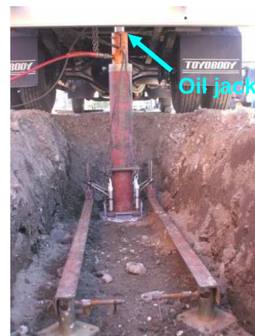
Photo 3 Static plate load test on Plate No.1
