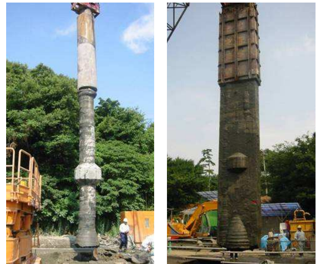
(a) Nodular cast-in-place concrete pile
