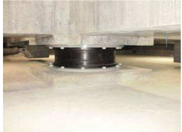
Photo 4 Laminated rubber bearings
