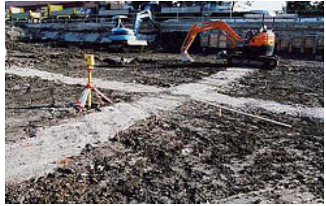
Photo 2 Grid-form soil-cement walls at the foundation level
