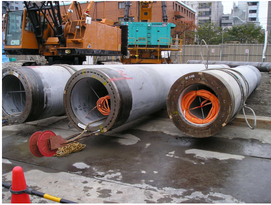
Photo 5 Instrumented PHC piles
