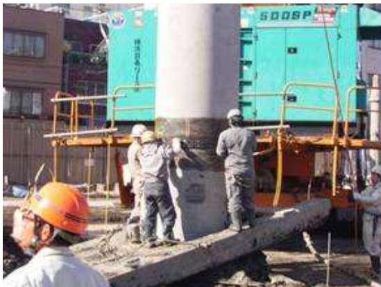
Photo 6 Construction of PHC piles (1.2m in diameter)
