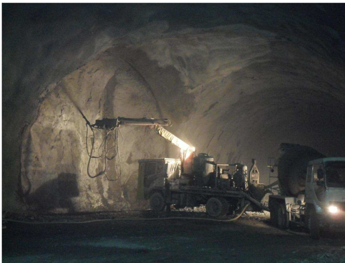
Figure 38 Shotcrete placements after the blasting
