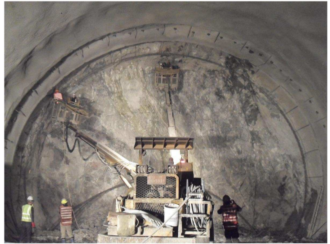
Figure 40 Steel rib (Lattice girder) installations
