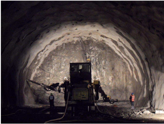
Figure 37 Drilling works for the blasting
