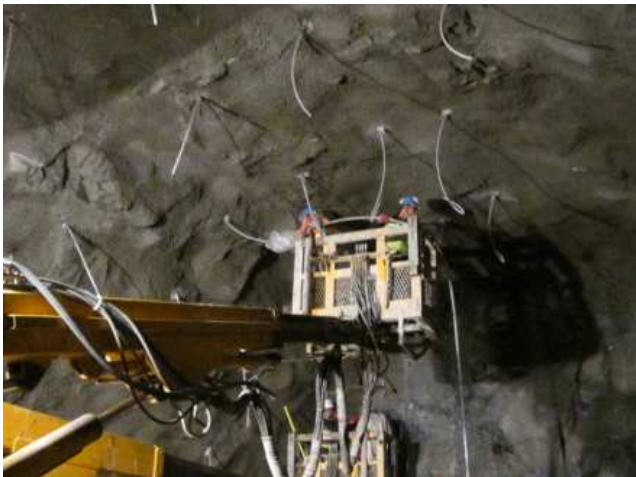
Figure 39 Rock bolt installations
