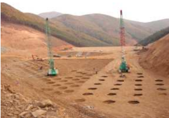
Figure 2. Scene of dynamic compaction
