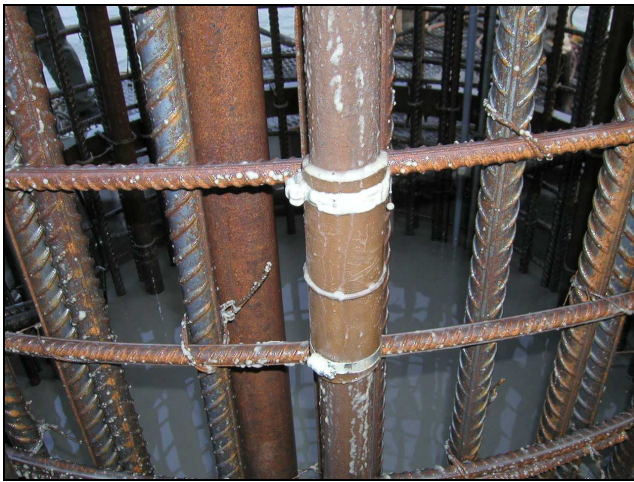
Figure 3. Fixture of TAM pipe on Pile Cage
