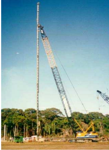
Figure 7. A 50m-vertical drain installation at Miri
