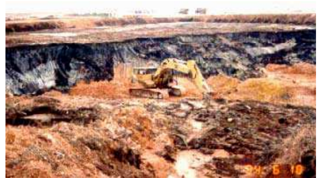
Figure 1. Excavation and replacement of unsuitable materials
