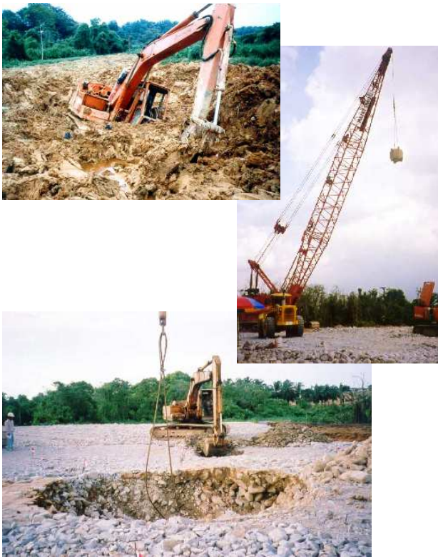
Figure 28. Site condition before treatment (top); 300 ton.m DR rig (middle) and 3.5m diameter DR rock column (bottom) at Senai.
