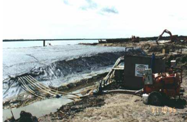
Figure 12. Vacuum consolidation for the New Kuching Deepwater Port at Kg. Senari, Sarawak
