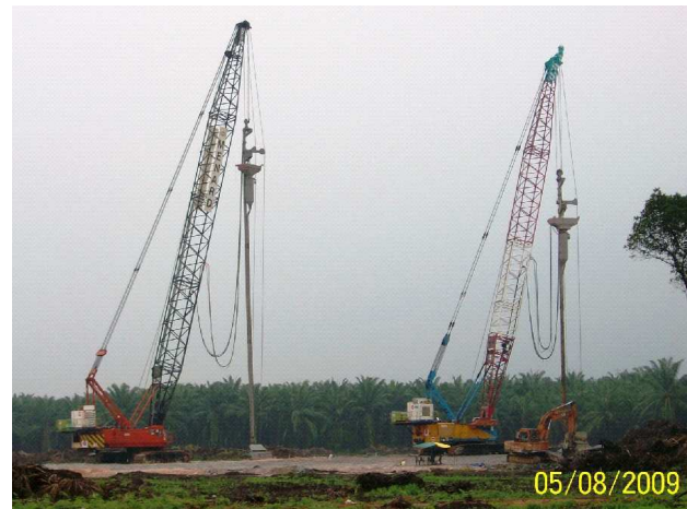
Figure 26. Dry bottom feed stone column installation at SKVE
