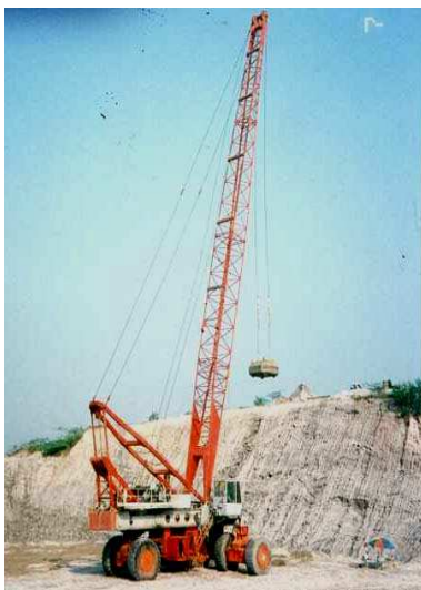
Figure 16. Hecto 750-ton.m DC rig used in Shah Alam Expressway
