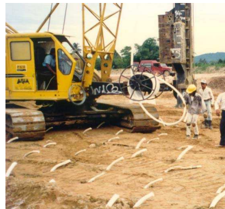
Figure 4. Installation of cylindrical vertical drains in Ipoh for the North-South Expressway
