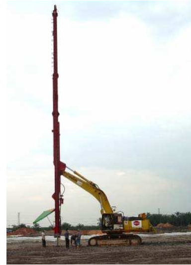
Figure 8. Installation of vertical drains using hydraulic rig.
