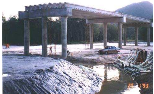
Figure 10. Vacuum consolidation for the North-South Expressway in Ipoh
