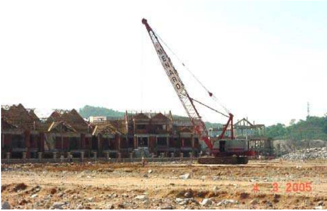
Figure 15. Dynamic compaction at Bandar Menjalara for double storey houses on non-engineered filled ground.
