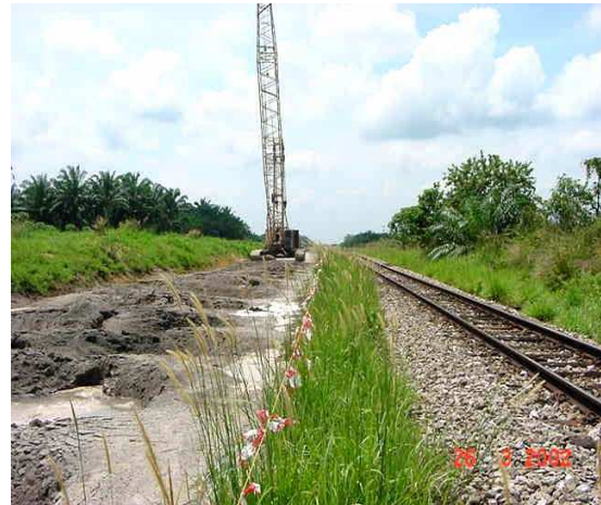
Figure 17. SVC using dynamic compaction at Bidor-Kampar for the Rawang – Ipoh Double Tracking project
