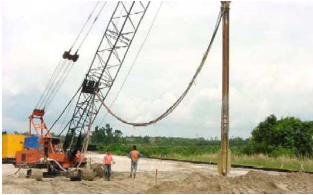
Figure 19. Electric vibroflot for sand compaction
