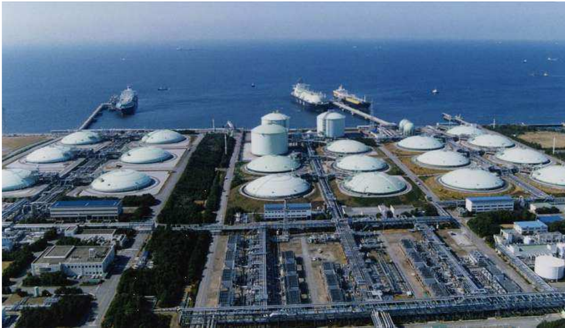
Figure 35. Underground LNG tank at Sodegaura, Chiba, Japan
