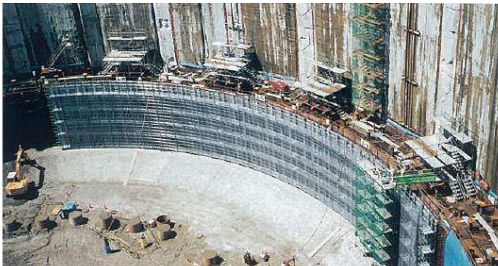
Figure 51. Installation of a block hoop at the depth of -28m
