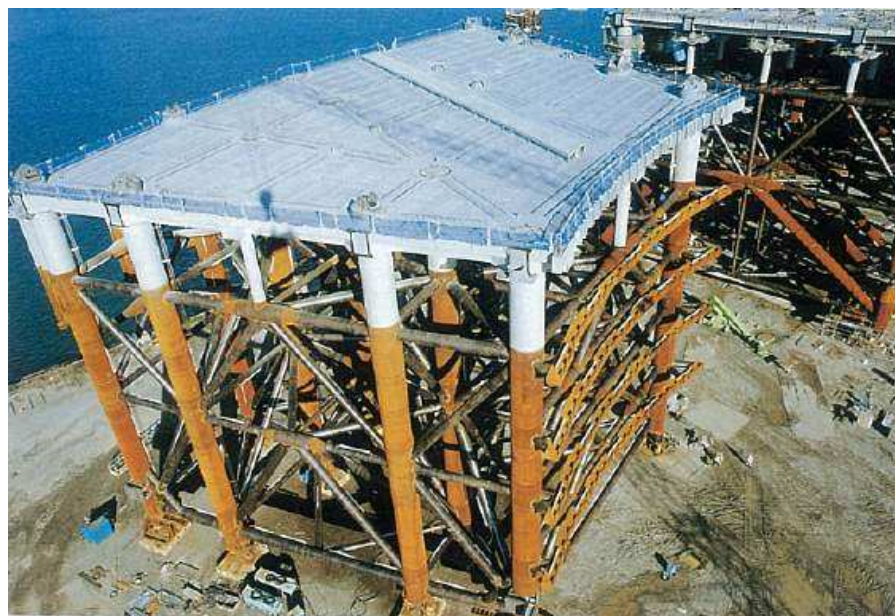
Figure 47. Unit of jacket frame sitting on the assembling yard
