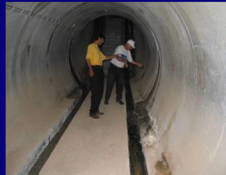
Figure 18. Keddara dam-cracks observed at the crest
