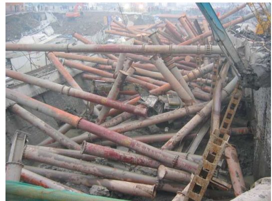
Figure 14 The messy struts after the collapse
