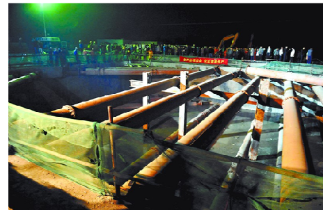
Figure 19 Pipe struts and their vertical support structure
