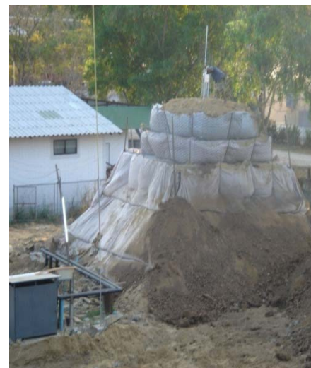
Figure 17 Use of geogrid, geotextile, and sand gabion blocks for increasing the slope of embankment (Pothiraksanon et al., 2010)
