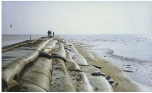
Figure 8 Dike constructed using clay slurry filled geosynthetic mattresses (Yan and Chu, 2010)
