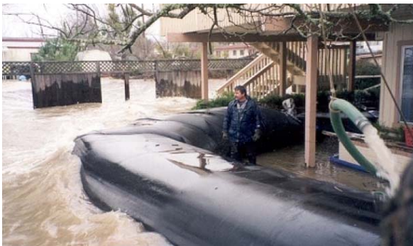
Figure 1 Geosynthetic tubes used for flood control (Howard and Trainer, 2011)
