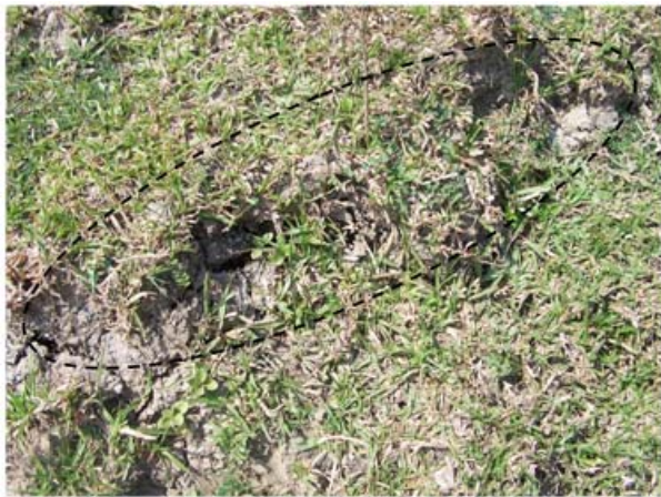
Figure 2 Close view of the slope along Tamluk Digha railway embankment (NTPC report, 2008)
