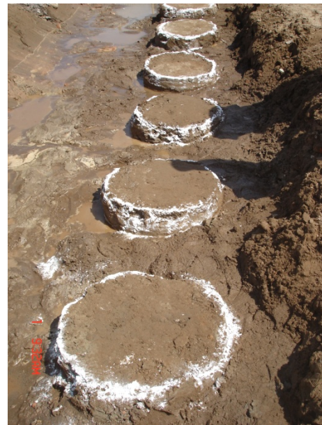
Figure 4 Surface exposure of cement mixed column
