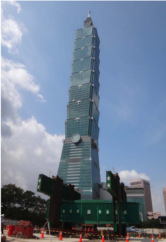
Figure 3 Photo of test C1 Shaft
