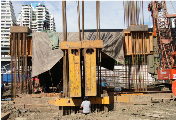
Figure 5 Photo of barrette pile test
