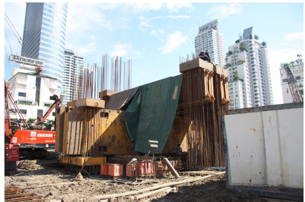
Figure 4 Photo of barrette pile test
