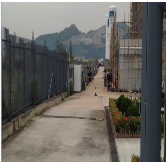
Figure 7 Subsidence of more than one metre
