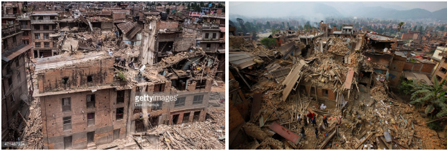
Figure 21 Damages of superstructures (globalnews.ca)
