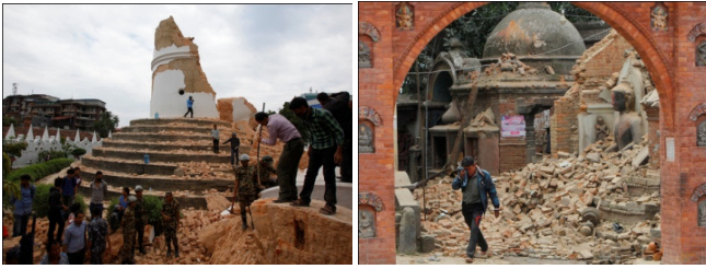
Figure 20 Damages of some historical places (National Post News)
