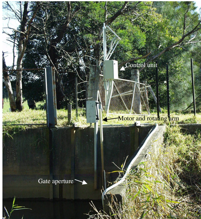
Figure 5 Modified two-way floodgate (Photo courtesy: Glamore (2003))
