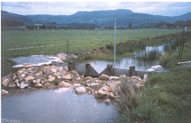
Figure 2 V-notch weir (after Banasiak (2004))
