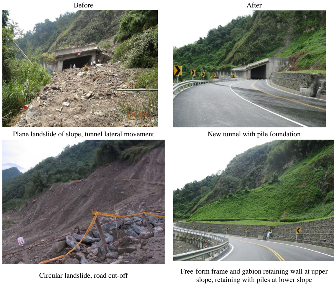
Figure 13 Before and after Photos at Mileage 59.1k of Alishan Route 18
