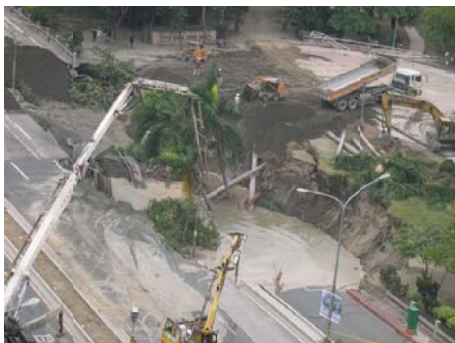
Figure 12 The large sinkhole on the south side and emergency backfill works in progress (daytime of December 5th, 2005)
