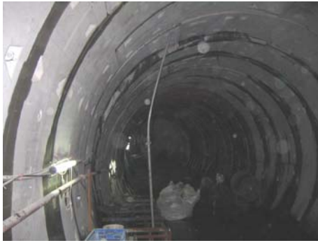
Figure 9 Serious water inflow and dislocation of lining segments inside the up-track tunnel (6:50pm, December 4th, 2005)
