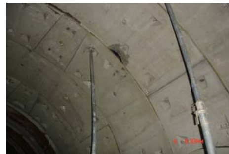
Figure 8 Concrete chunks detached from the ring segments of the up-track tunnel (6:30pm, December 4th, 2005)
