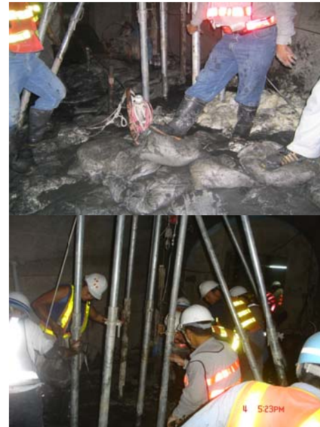
Figure 7 Effort made to seal the top of the sump (5:23pm, December 4th, 2005)
