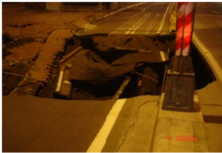
Figure 10 Sinkhole appeared on the ground above the up-track tunnel (10:05pm, December 4th, 2005)
