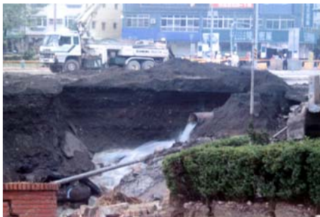
Figure 11 Rupture of the water main (morning of December 5th, 2005)
