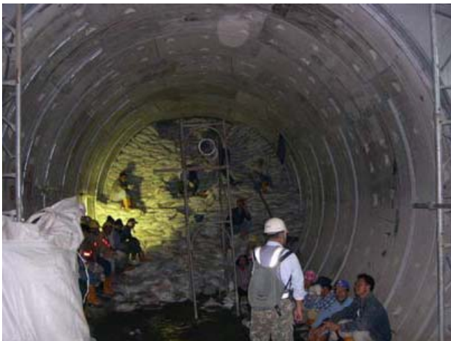
Figure 16 Construction of double layer wall at O7 station side
