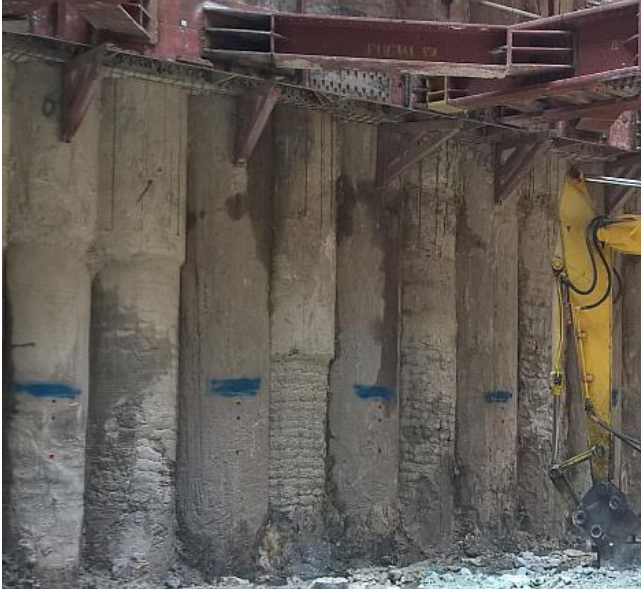
Figure 25 Section of SBP at approximately 25m bgl between cased and uncased SBP.
