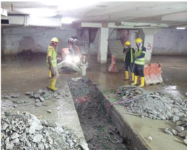
Figure 18 Pre-cutting of existing basement slab, to enable D-wall work to proceed at Pasar Seni Station
