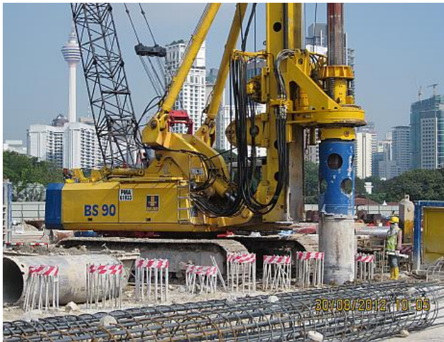
Figure 21 Boring works for Secant Bored Piles wall
