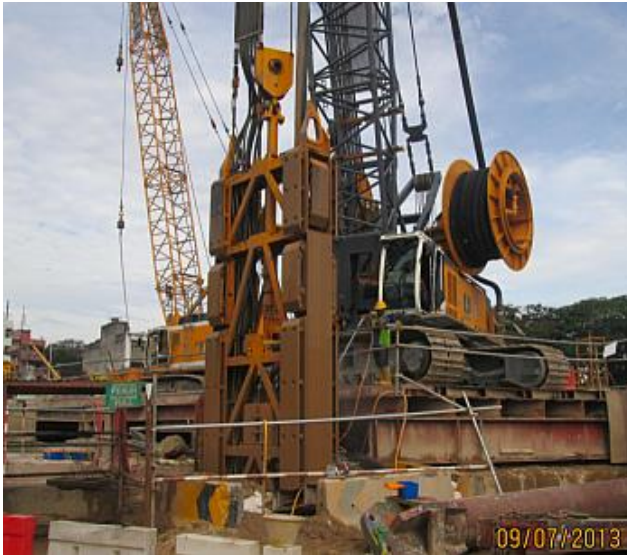
Figure 17 'Trench Cutter' D-wall machine at Pasar Seni Station sitting on temporary platform.
