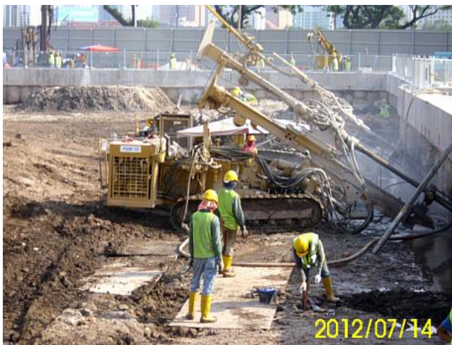
Figure 22 Installation of Temporary Ground Anchors for the SBP wall.
