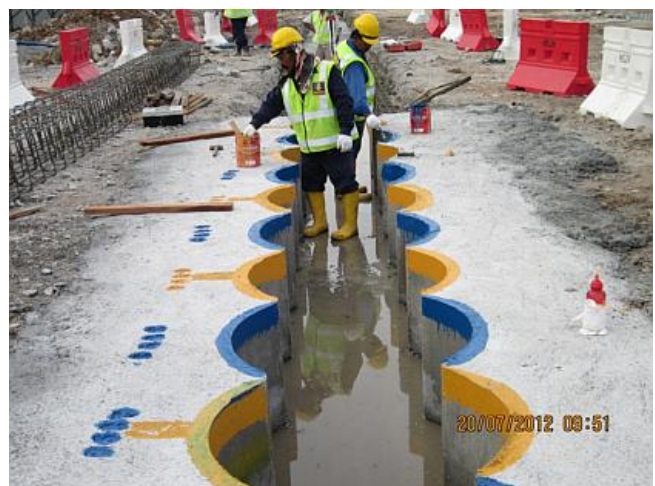
Figure 20 SBP Guide wall being prepared prior to drilling works
