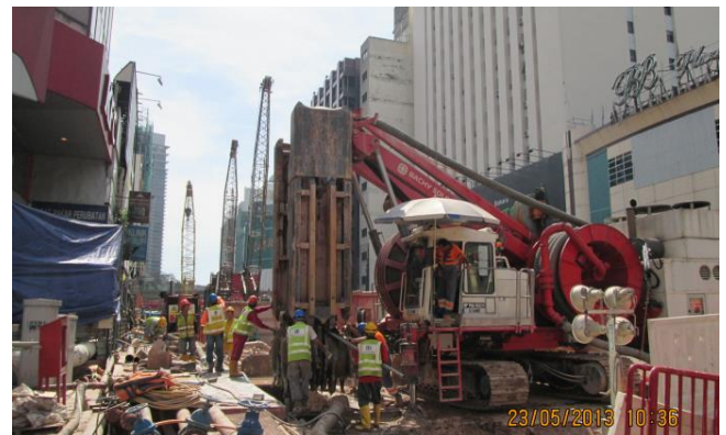
Figure 16 Low Headroom 'Hydrofraise' D-wall machine at Bukit Bintang Station
