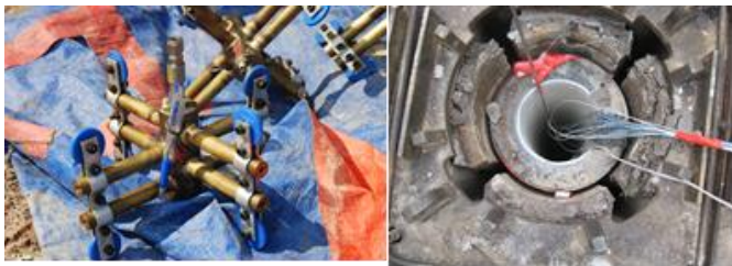
Figure 19 Installation of Glostrex Instrumentation System for the Test Pile
