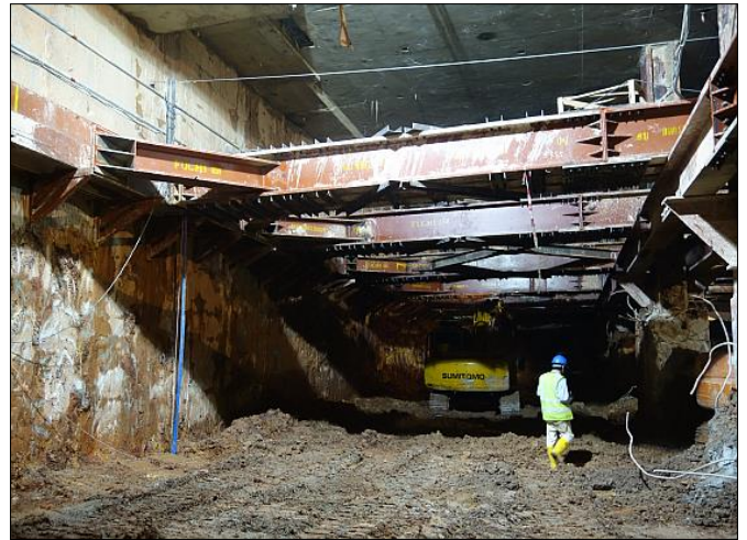
Figure 20 Bukit Bintang Station, Top-up excavation in progress at the lower platform level.
