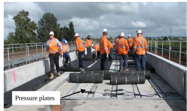
Figure 12(b) Location of Mudies Creek Bridge and Installation of shock mat
