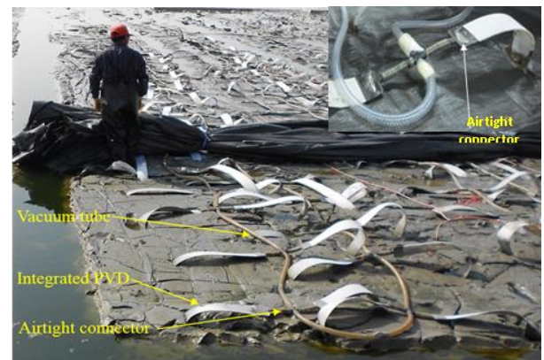
Figure 19 Connectors used to connect PVDs directly to the vacuum distribution pipes (after Wang et al. 2016)
