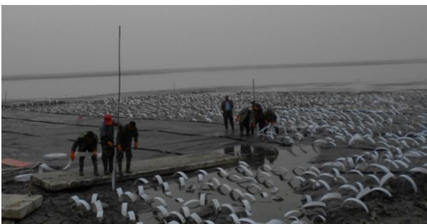
Figure 17 Installation of PVDs from a platform made of foam boards (after Wang et al. 2016)
