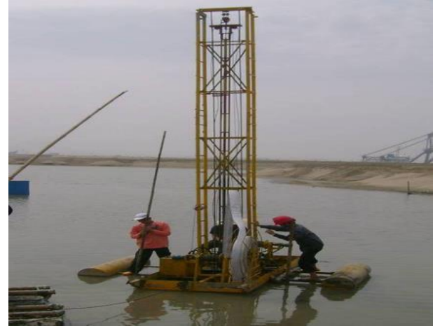
Figure 18 Floating vertical drain installation rig for installation of short drains (Courtesy of Yan S.W.)
