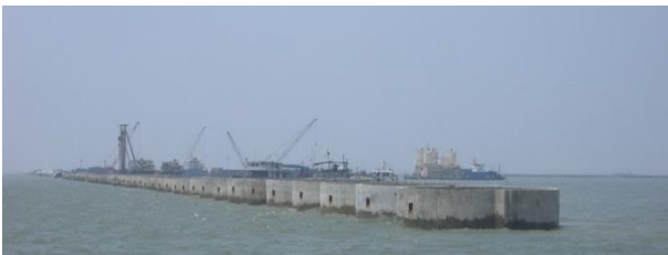
Figure 23 An offshore breakwater constructed using suction caissons (Chu et al. 2012)
