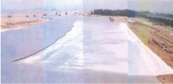
Figure 15 Installation of geotextile sheet for the slurry pond land reclamation project in Singapore (after Chu et al. 2009a)
