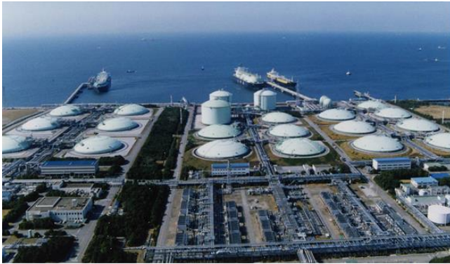
Figure 35 Underground LNG tank at Sodegaura, Chiba, Japan
