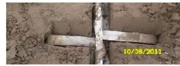
(a) Connection of PVDs to horizontal flexible pipe
