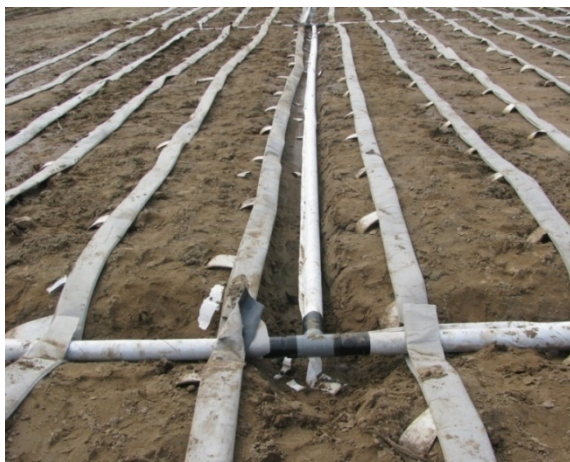
Figure 12 VCM-MB using airtight membrane and horizontal band drains (Long et al, 2011)
