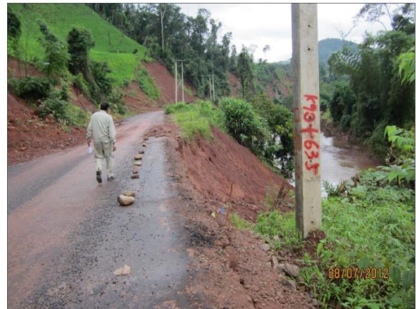
Figure 5 Erosion at the lower slopes due to river flooding causing slope failures in Phongsali Province, Northern Laos PDR
