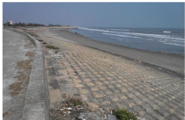
d) Concrete revetment
