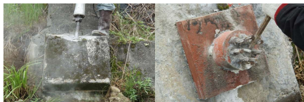
Figure 8 Remove the concrete protection cap of anchor head
