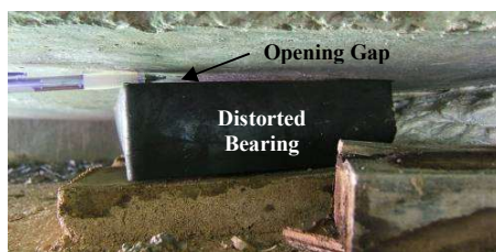
Figure 15 Shearing distortion of rubber bearing
