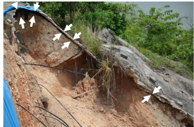
Figure 21 Gap Formation between Soil Nailed Slope and Shotcrete Facing
