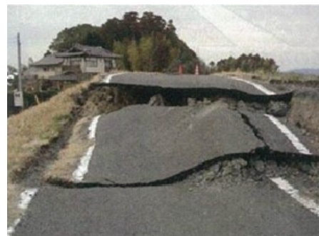
(a) River dyke failure
