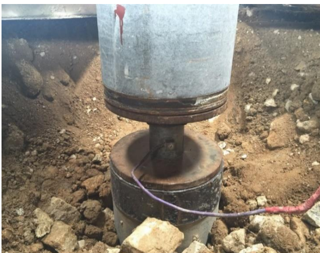
Figure 4 Site calibration of jack-in machine pressure gage with the use of load cell
