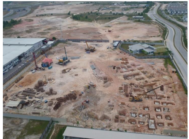
Figure 3 Example of jack-in pile construction site
