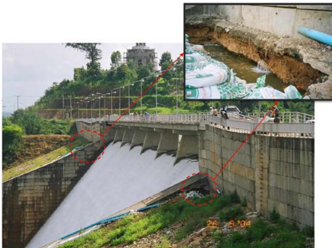
Figure 5 Leakage observed at the joint between RCC and earth fill dam; the differential settlement is clearly seen (Photo by RID)
