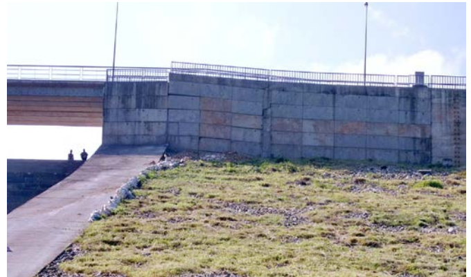
Figure 7 Elevation of RCC Block D and differential settlement at left bank (Photo by RID)
