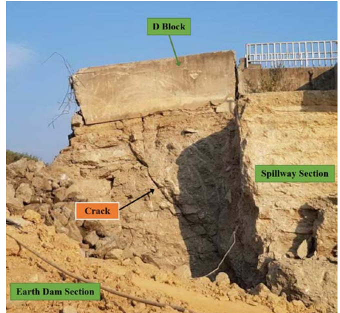
Figure 24 Crack appeared in the rehabilitation processes of Mae Suai Dam (2019)
