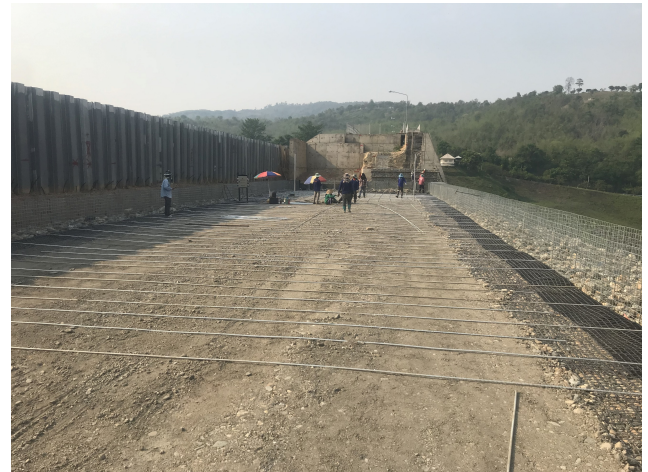
Figure 6 Rebar reinforcements installation
