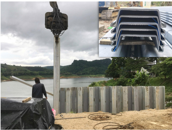
Figure 17 The hot-dipped galvanized steel sheet pile
