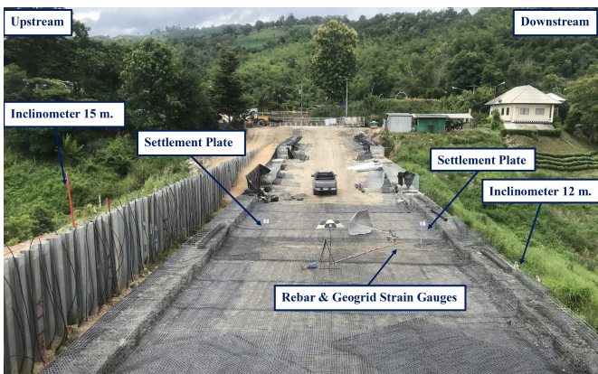
Figure 10 Geogrid installation and instrumentation of test section (left Bank)
