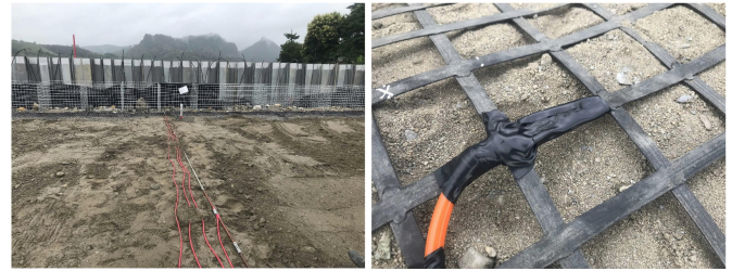
Figure 11 Rebar and Geogrid strain gauges installation (a) rebar strain gauges (b) geogrid strain gauges
