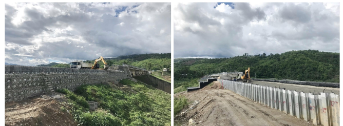
Figure 7 Construction of full scale MSE wall
