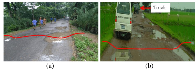
Figure 27 Water logging on the new pavement road. (a) Initial settlement and (b) settlement and wide spread pot holes.
