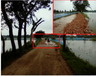
Figure 23 A portion of road settled.
