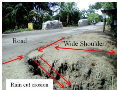
Figure 18 Rain cut erosion in shoulder without vegetation
