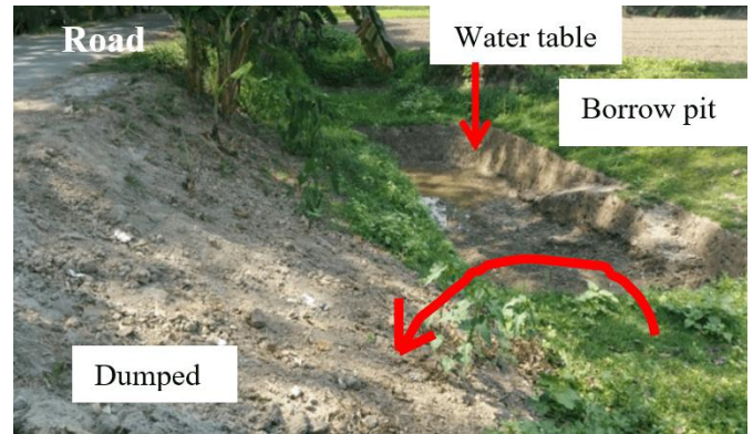
Figure 9 Borrow pit was at the toe of the road. (Location: Babubazar, Barishal).
