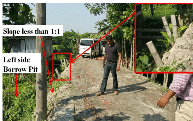
Figure 8 Steep side slope of rural roads in the study area (Location: Uttarpara, Uzirpara, Barishal).
