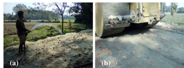
Figure 6 (a) Mixed brick chips and sand (1:1) in Sub-base and watering before rolling and (b) after rolling.
