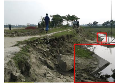
Figure 26 Palisading failed.
