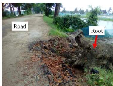
Figure 20 Uplifted tree damaged the road.
