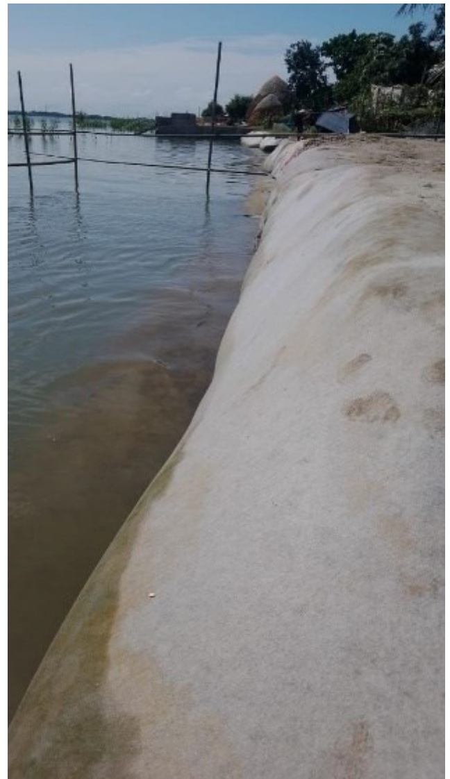
Figure 14 (a) Wrap-faced wall after flooding
