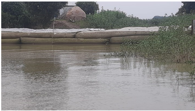
Figure 14 (b) Wrap-faced wall after flooding
