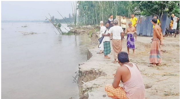
Figure 11 Typical embankment failure in Bangladesh
