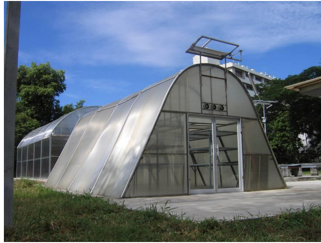
Fig. 1 Pictorial view of the parabolic greenhouse solar dryer.
