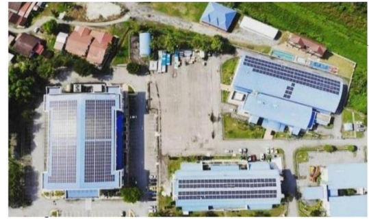
Fig. 2 The existing IHL grid-connected solar PV systems.
