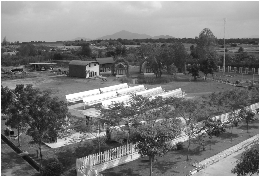
Fig 4. View on the station with solar field and boiler house
