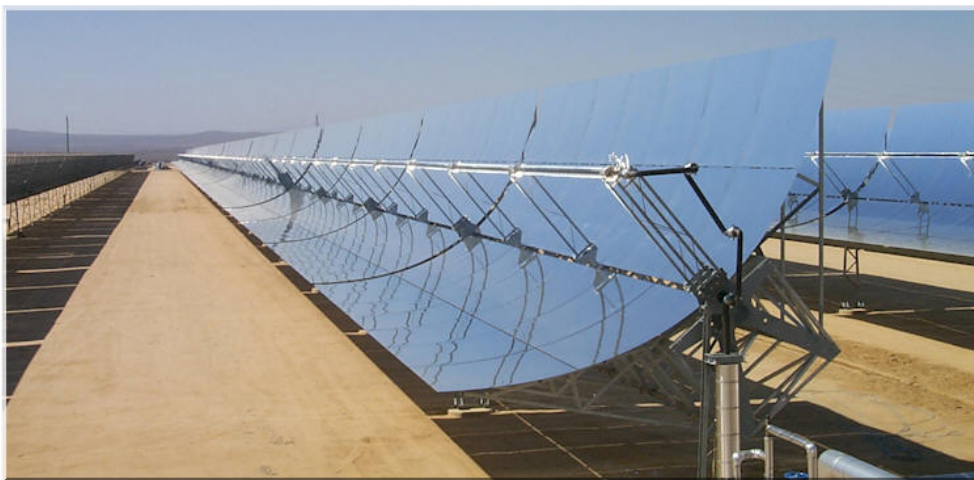
Fig.1 Parabolic trough collectors field at the Kramer Junction, California [9].
