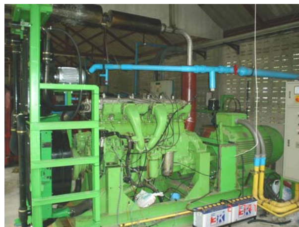
Fig 6. A picture of the assembled biogas generator.
