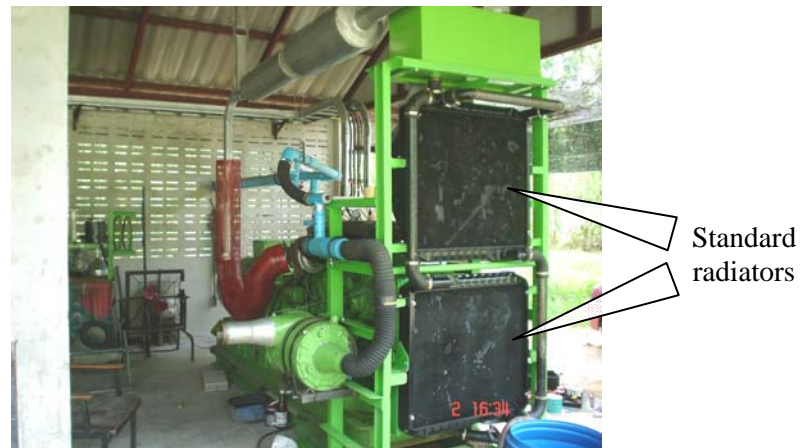
Fig 5. A picture of the two standard radiators of the biogas generator.
