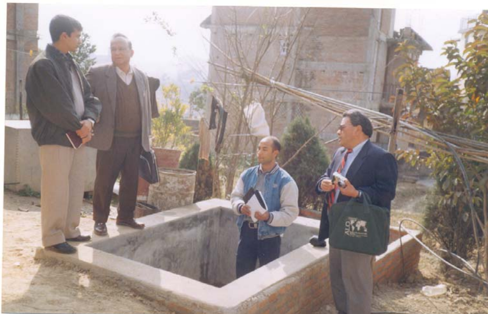
Fig. 2 Plant under Construction and a Visit by Professors/ Supervisors
