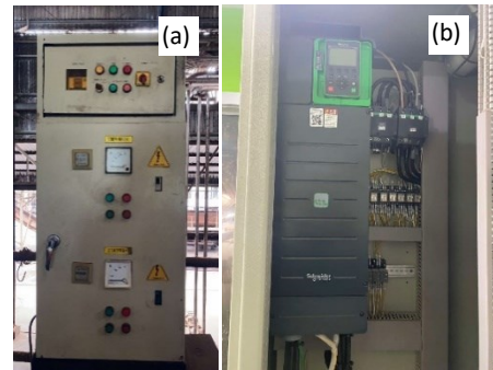
Fig. 5 (a) Before and (b) after installing inverters for motors.
