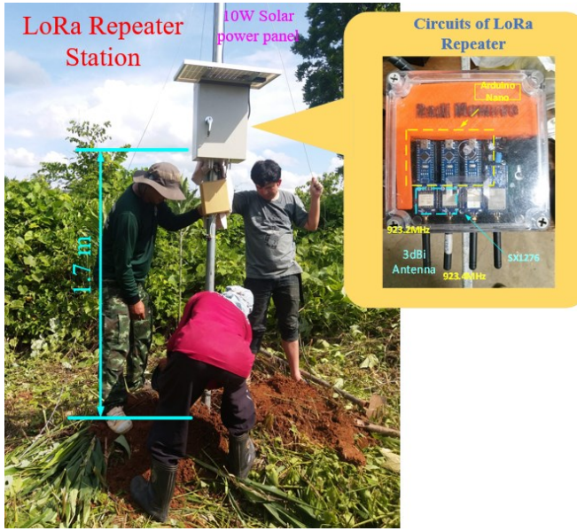
Fig. 8 The installation location of the LoRa repeater.
