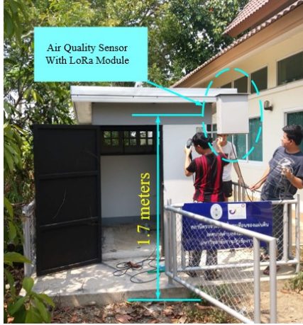
Fig. 4 The installation location of the LoRa node air quality station.
