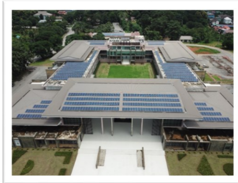
Fig. 3 Showing the solar PV rooftop installed 500 kWp at Chiangrai Rajabhat University.
