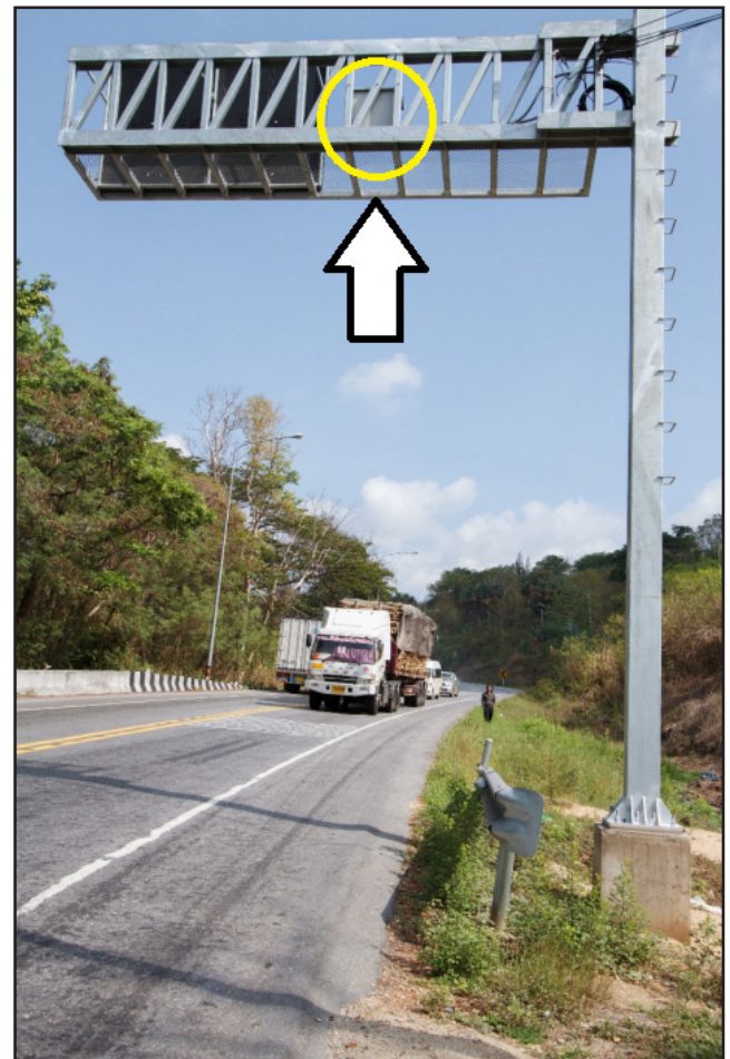
Figure 1. Display how the radar traffic equipment is installed.
