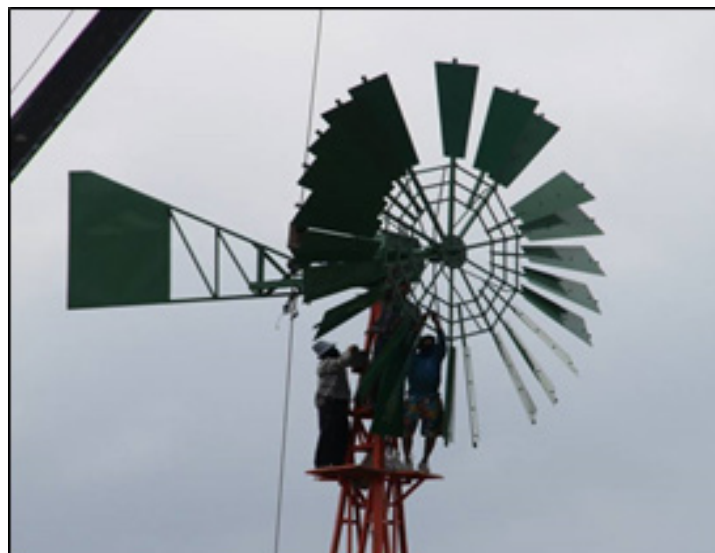
Figure 8. Installation of the multi-blade wind turbine
